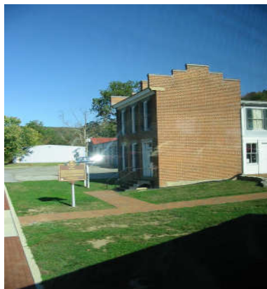
Parker House –side view
